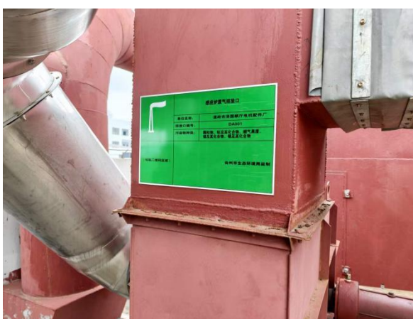
DA001 感应炉废气排气筒
